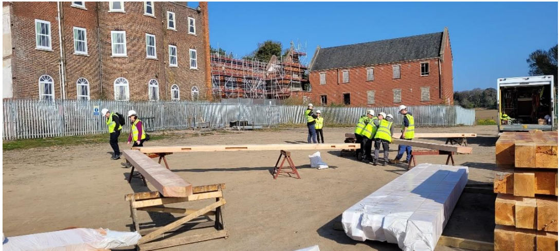
Chapel Roof repairs underway March 2022 – CORA Main Hall on the left
