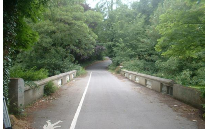
Causeway between the two lakes – WM 2004
